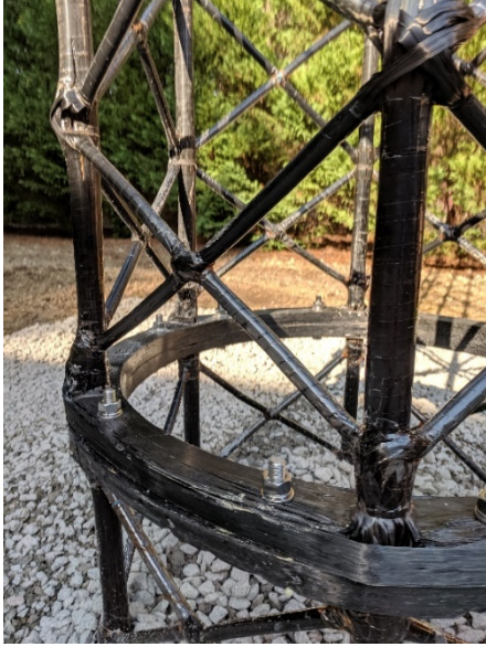
Figure 4. Photographs of IsoTruss connections. Towers (left) use bolted connections, while bikes (right) use joints that are manufactured separately and then attached.
